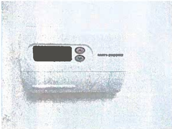
Photo #19 Typical wall mounted electronic thermostat.
