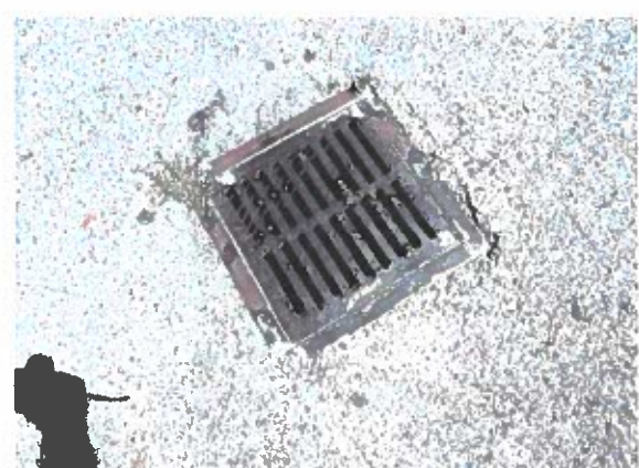
Photo #38 Typical storm water manhole.
