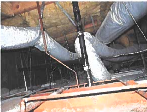
Photo #28 Typical view of above ceiling shows some of the plumbing piping and flexible ducts.
