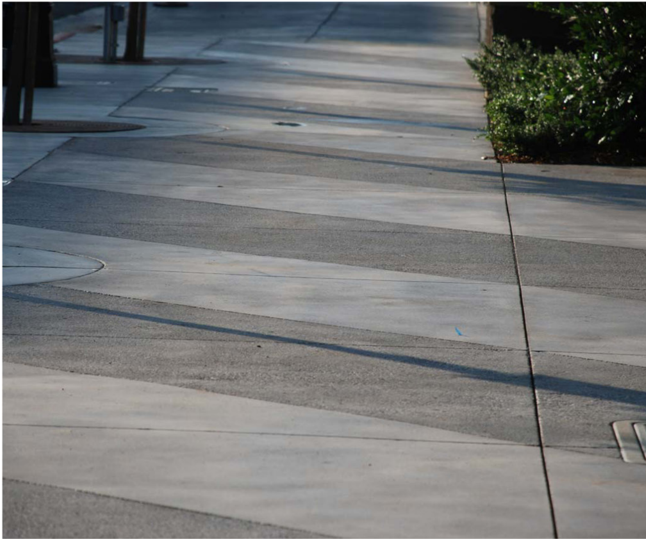
Concrete Paving with Alternating Concrete Finish
