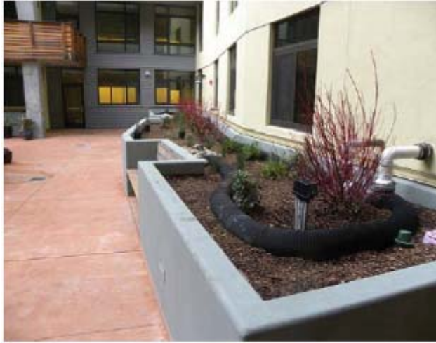
Figure 6-12: Half-buried, perforated flexible pipe serves as a flow spreader to distribute stormwater evenly throughout a long flow-through planter in Emeryville (Source: GreenGrid/Weston Solutions).
