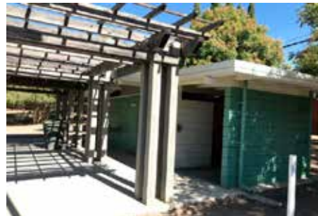
#20 AUGUSTINE PARK RESTROOM
