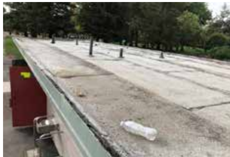
#67 MURPHY PARK ROOF
