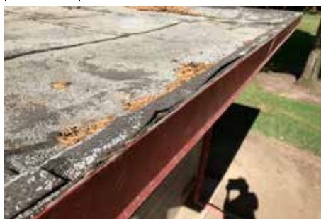
#71 SINNOTT PARK ROOF, MODIFIED BITUMINOUS
