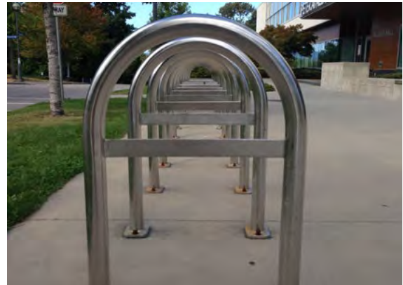
INVERTED U RACKS PROVIDE A MORE SECURE AND STABLE OPTION FOR SHORT TERM BIKE STORAGE.
