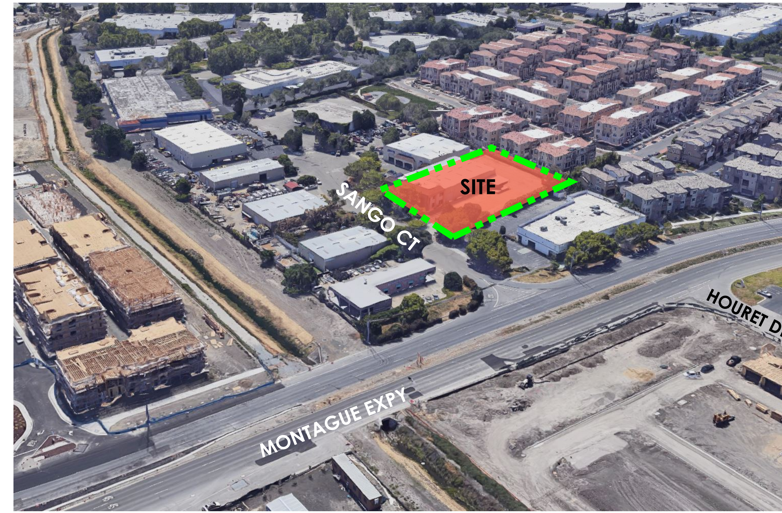
AERIAL VIEW LOOKING SOUTHEAST
