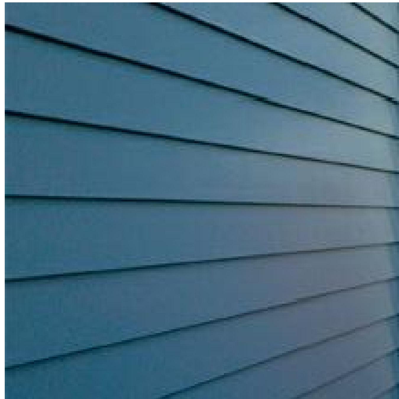
EXAMPLE: CEMENTITIOUS LAP SIDING
