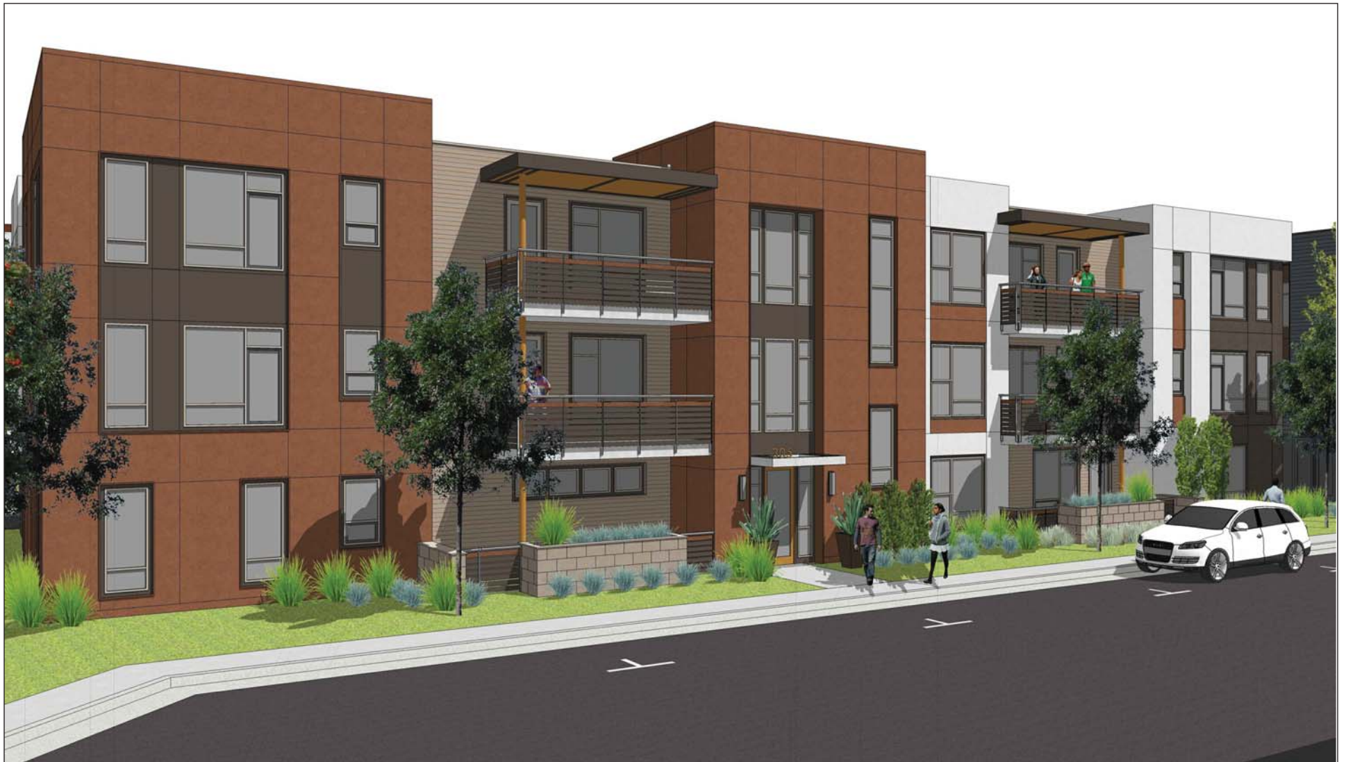
View of the Townhouses from Internal Road
