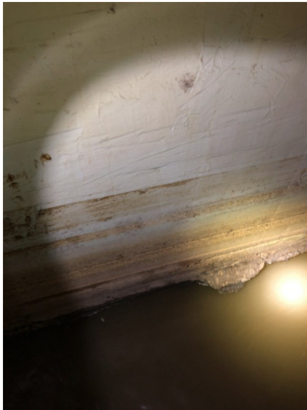
Dirt on steel not corrosion
