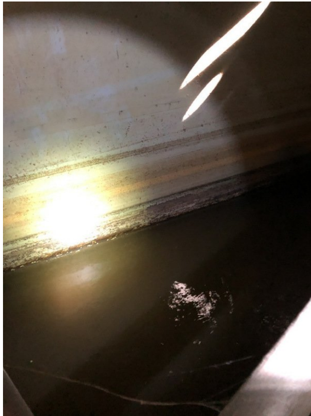
Eroding of coating and concrete, color change at bottom
