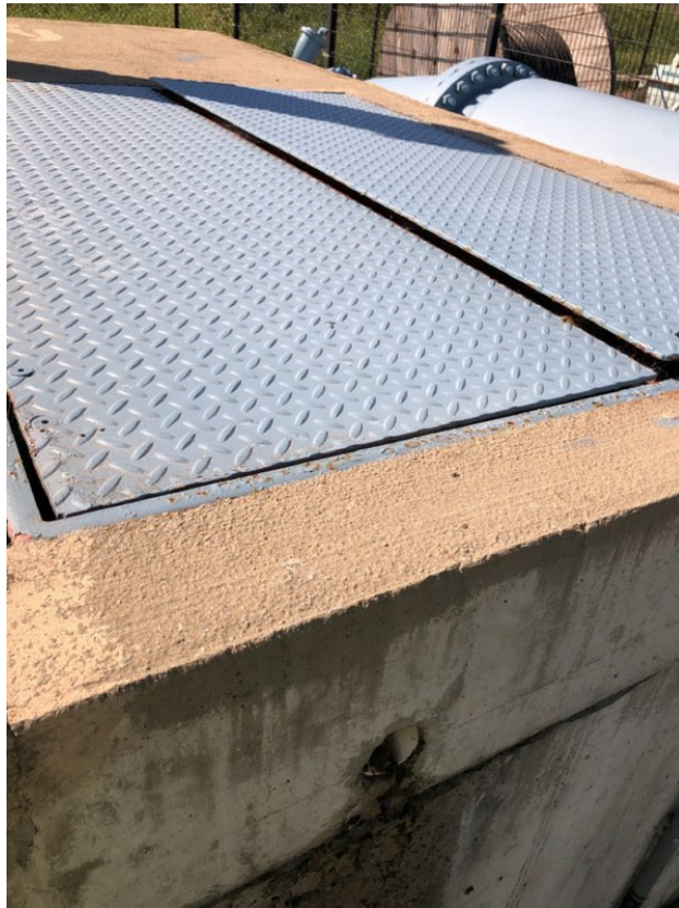
Corroded lid
