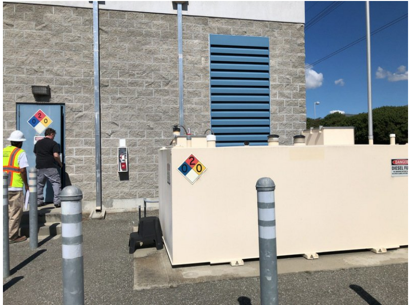
Right side of building
