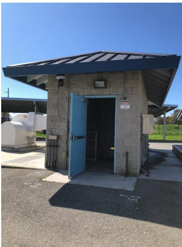
Building on top of wet well, entrance to wet well
