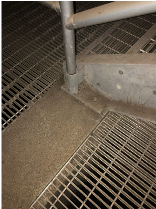
Stair knee brace connection
