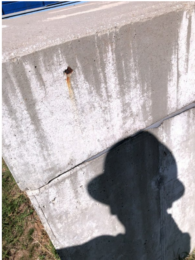
Exposed rebar
