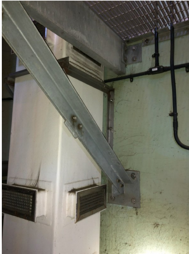
Stair knee brace connection
