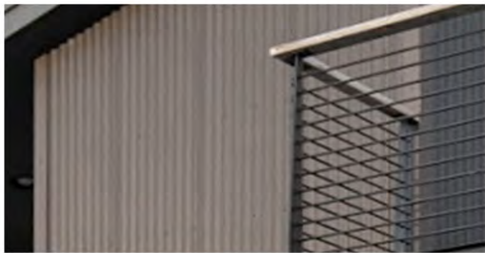
1 VERTICAL SIDING VERTICAL FIBER CEMENT SIDING
