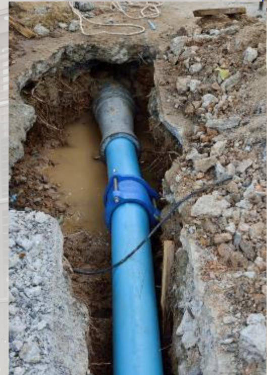
Replacement/Rehab of Aging Pipelines
