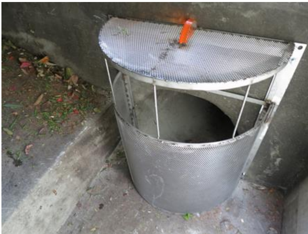
Stormtek ST3-G Connector Pipe Screen Trash Capture Device
