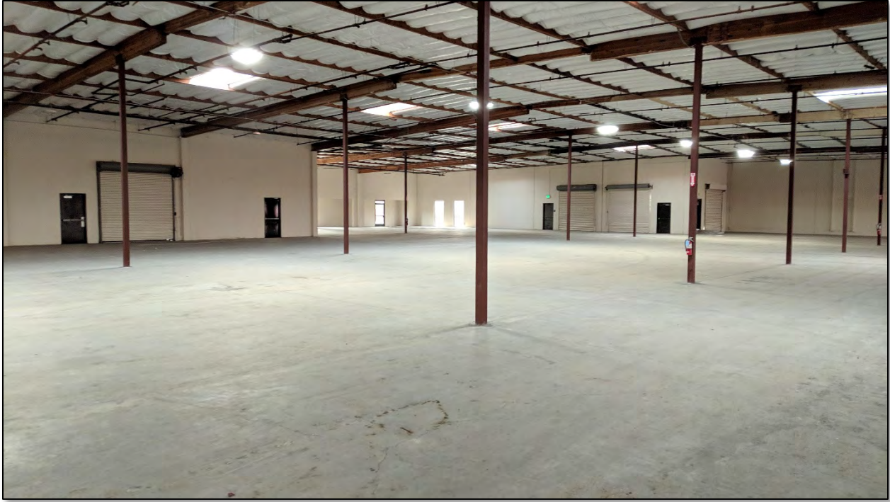
View of the warehouse portion of the building located on the subject property (typical)
