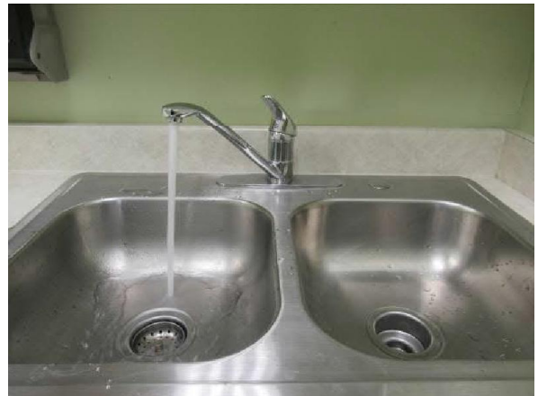
Photo #22 View of typical sink hot/cold water testing.
