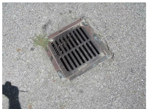
Photo #38 Typical storm water manhole.
