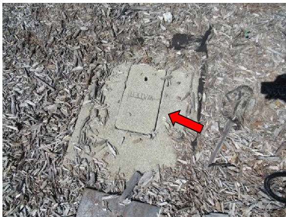
Photo #37 View of the water meter manhole.
