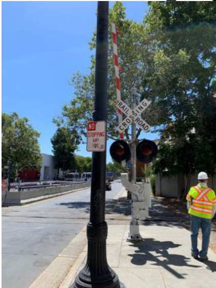
11_N 1 St Southbound Gate_facing S.jpg
