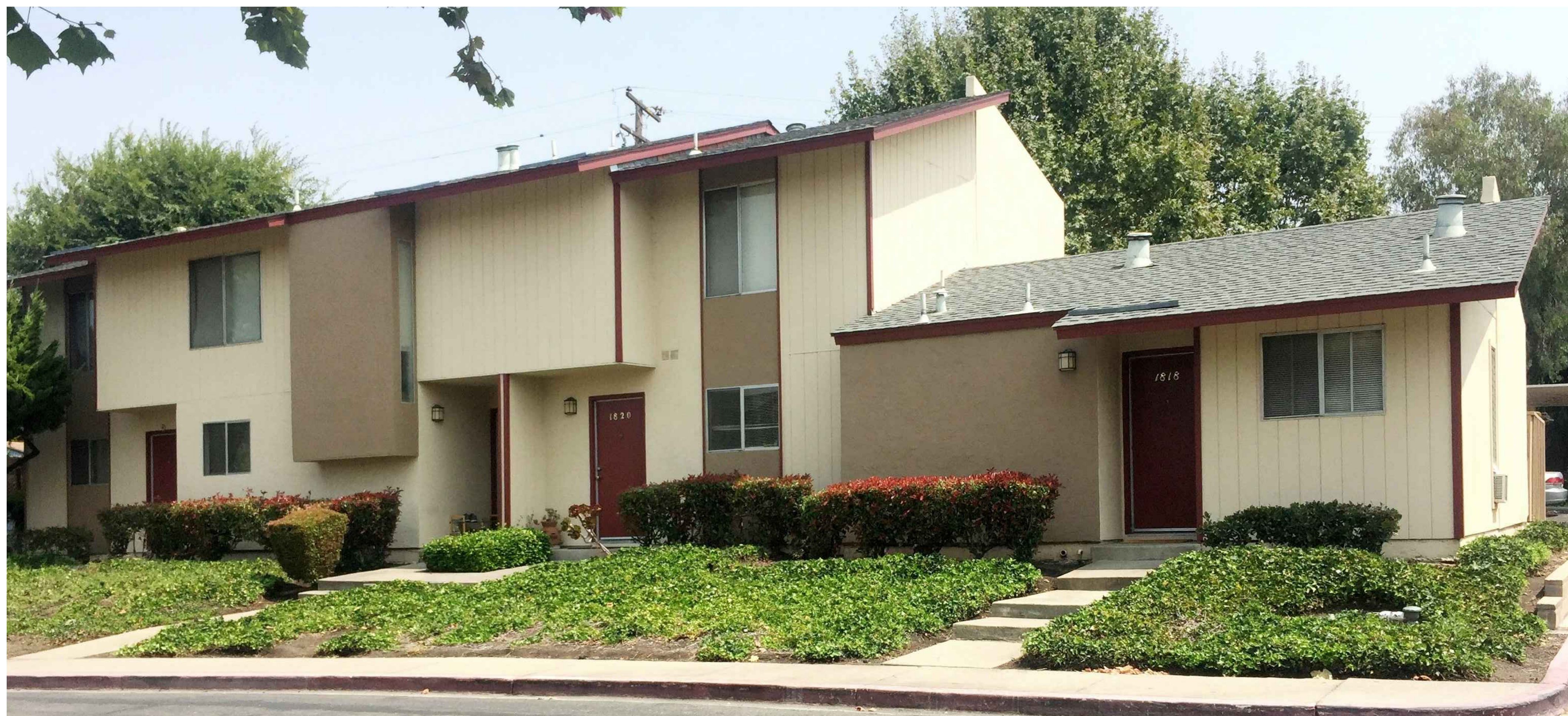
COLOR SCHEME OF TYPICAL EXISTING BUILDING
