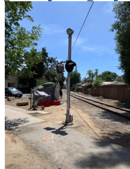
28_N 6 St Signal Pole_facing S.jpg
