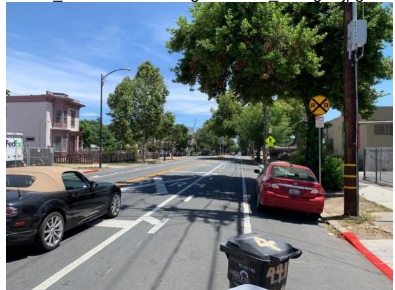
20_N 4 St Railroad sign&W10-2_facing S.jpg
