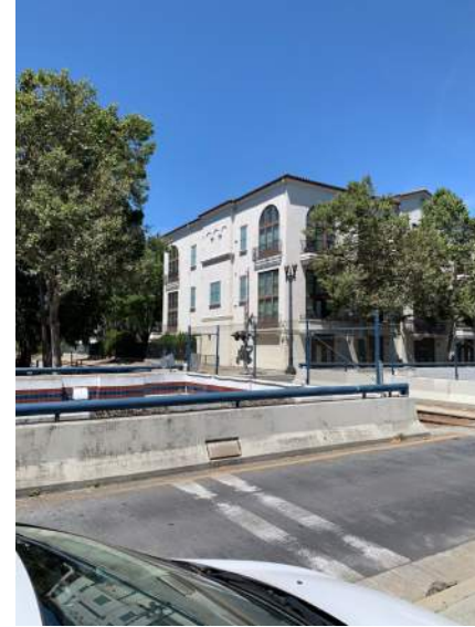
10_N 1 St Bridge_facing W.jpg
