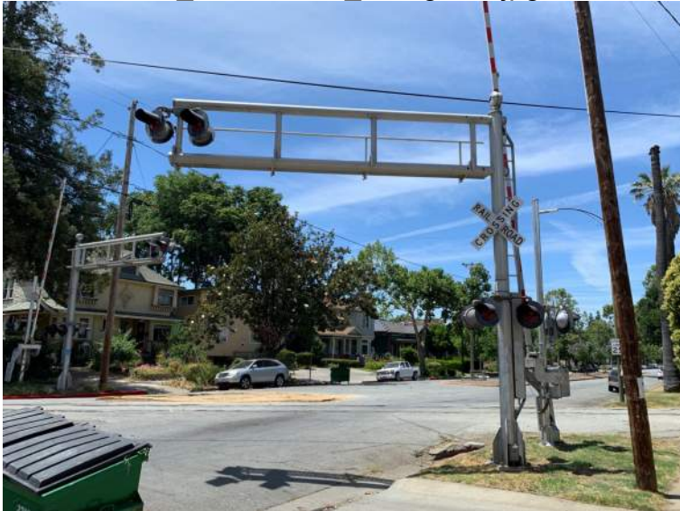
21_N 5 St Gate_facing NW.jpg
