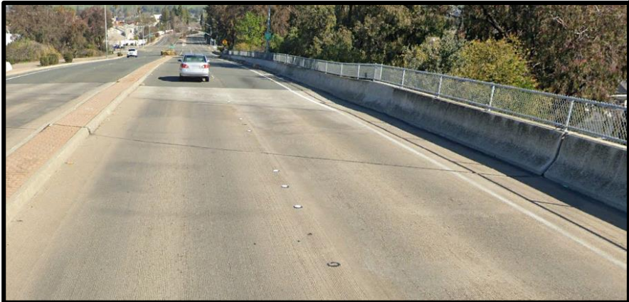
N Abel St over Railroad Tracks
