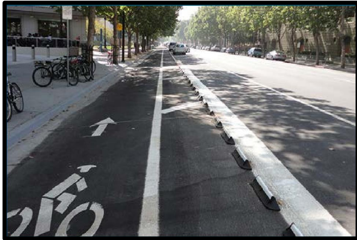
Class IV Separated Bikeway *No Existing Class IV Facilities within the City
