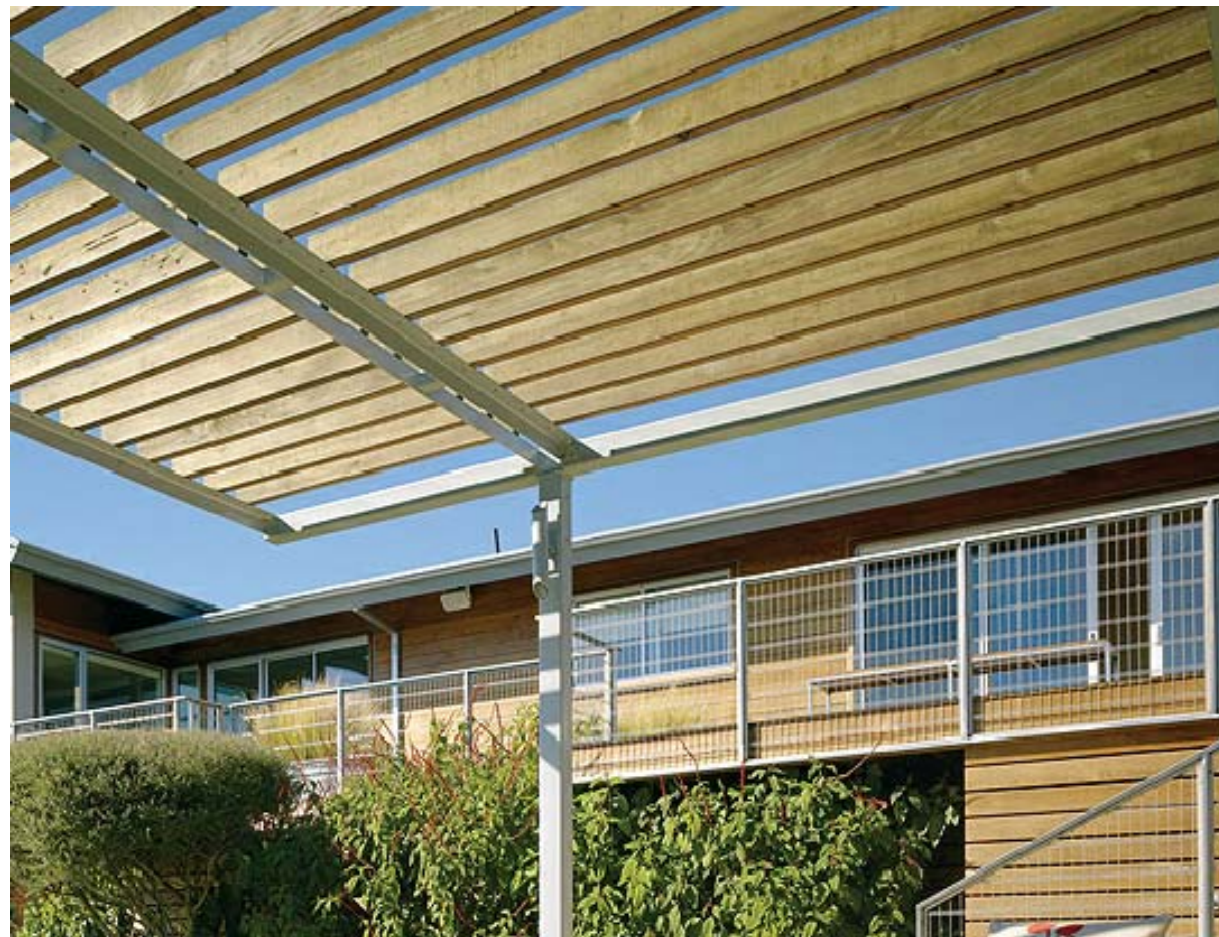
WOOD AND PAINTED STEEL PATIO TRELLIS | 6
