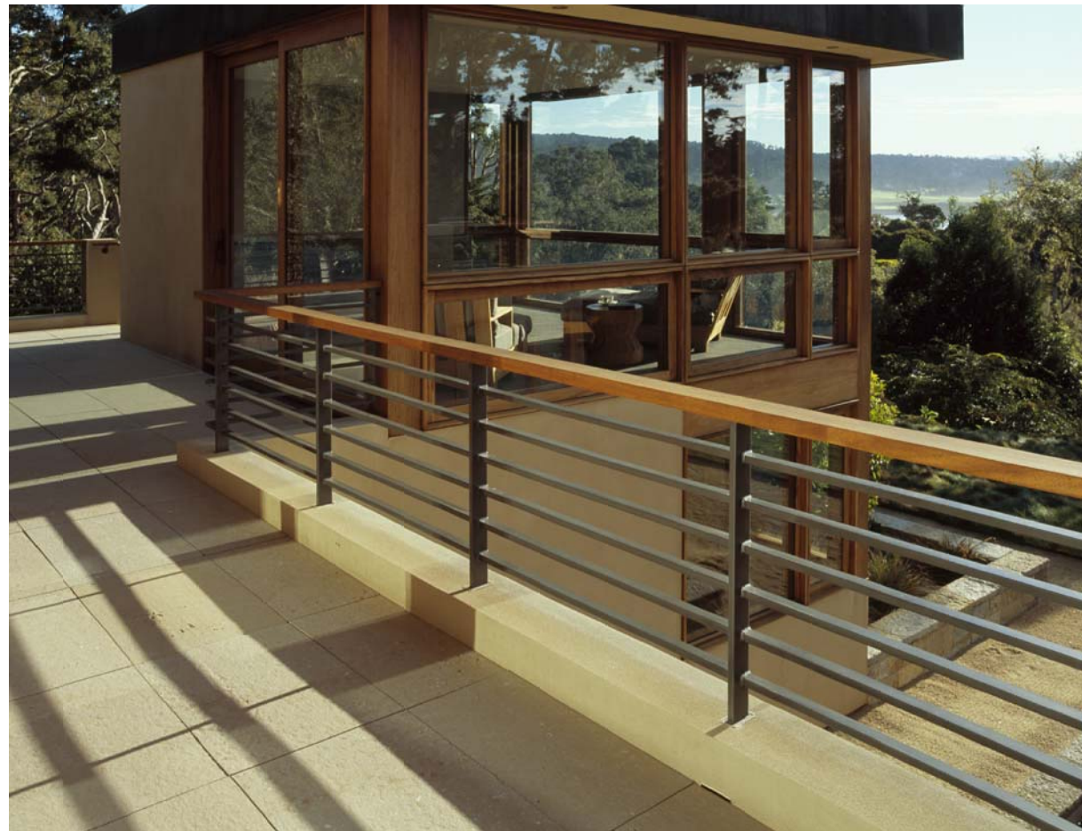
WOOD AND PAINTED STEEL GUARDRAILS | 7
