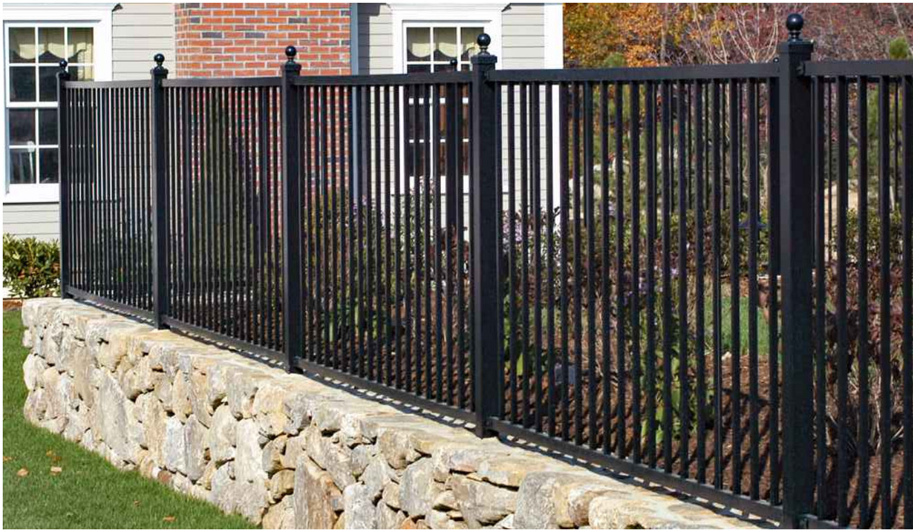
METAL FENCE ON RETAINING WALL
