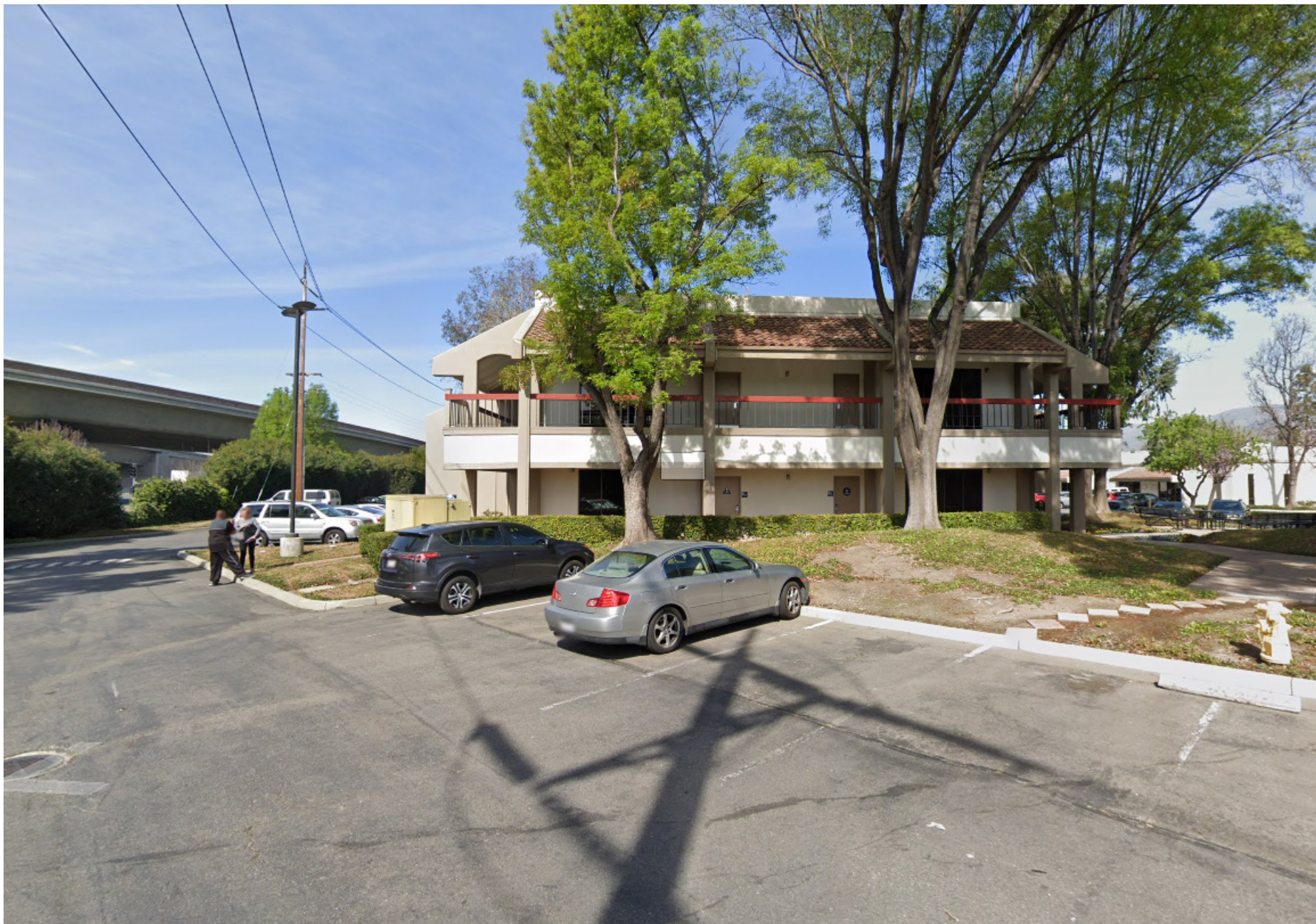
EXISTING SITE CONDITION - LOOKING NORTH 3
