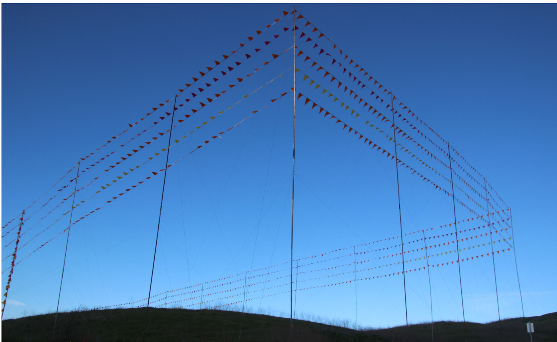
STORY POLES INSTALLED AT SETBACK LINES AND CONTINUED INTO CRESTLINE ZONE OF PROTECTION.
