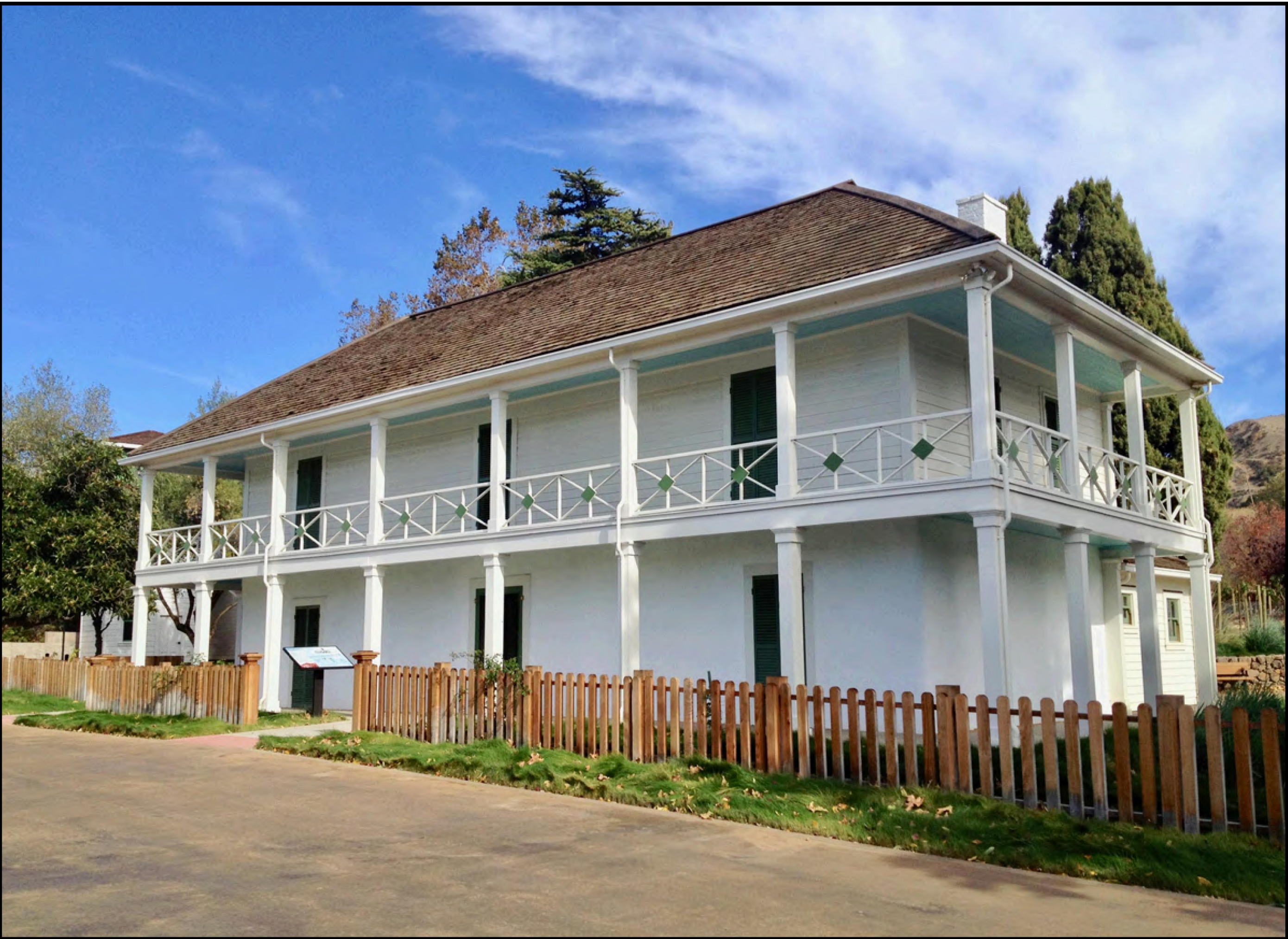
ALVISO ADOBE BUILDING
