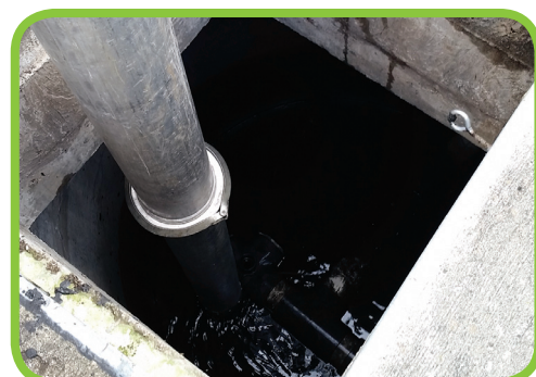
Jet Vactoring Through Access Hatch
