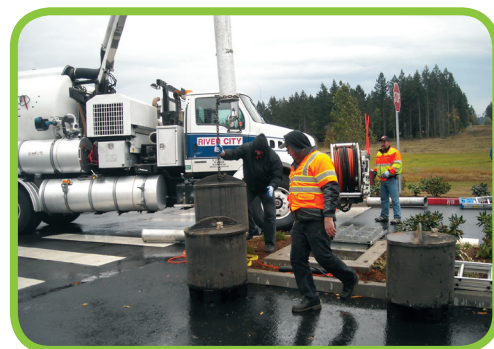
BayFilter System Cleanout
