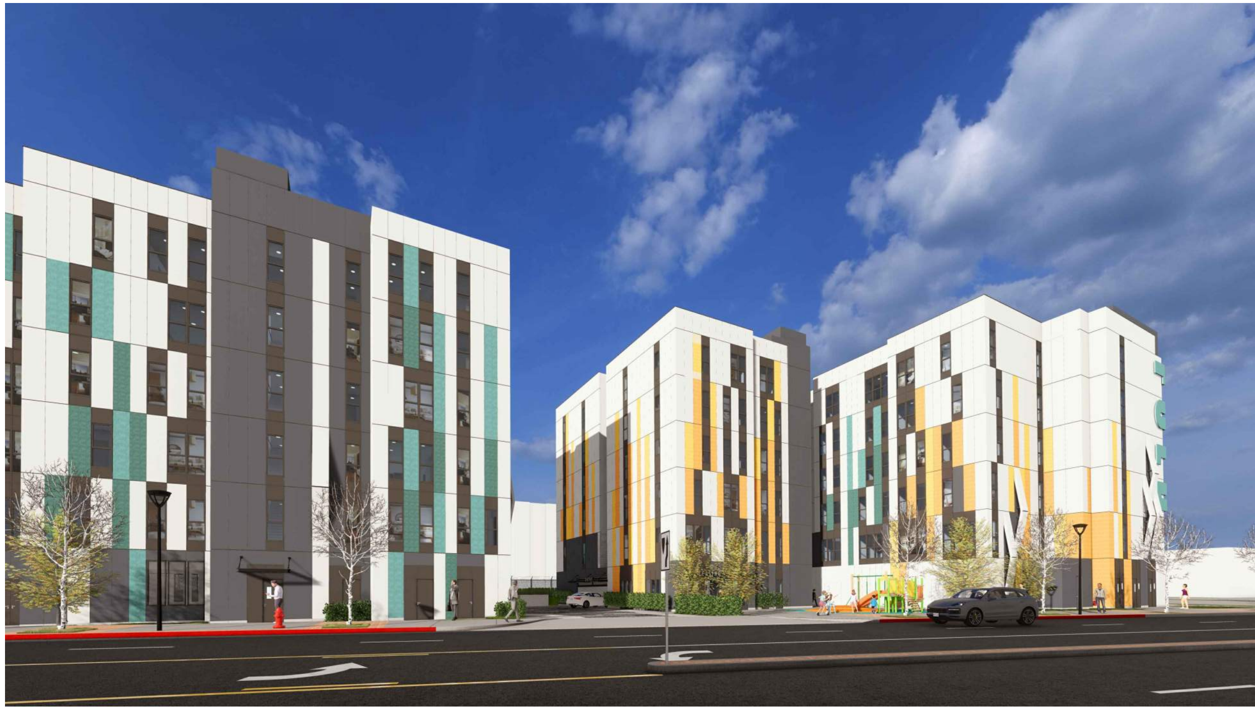
VIEW ON MAIN STREET LOOKING SOUTHEAST 2
