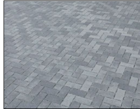
10 MIXED MEDIUM TO LIGHT GREY PERVIOUS PAVERS
