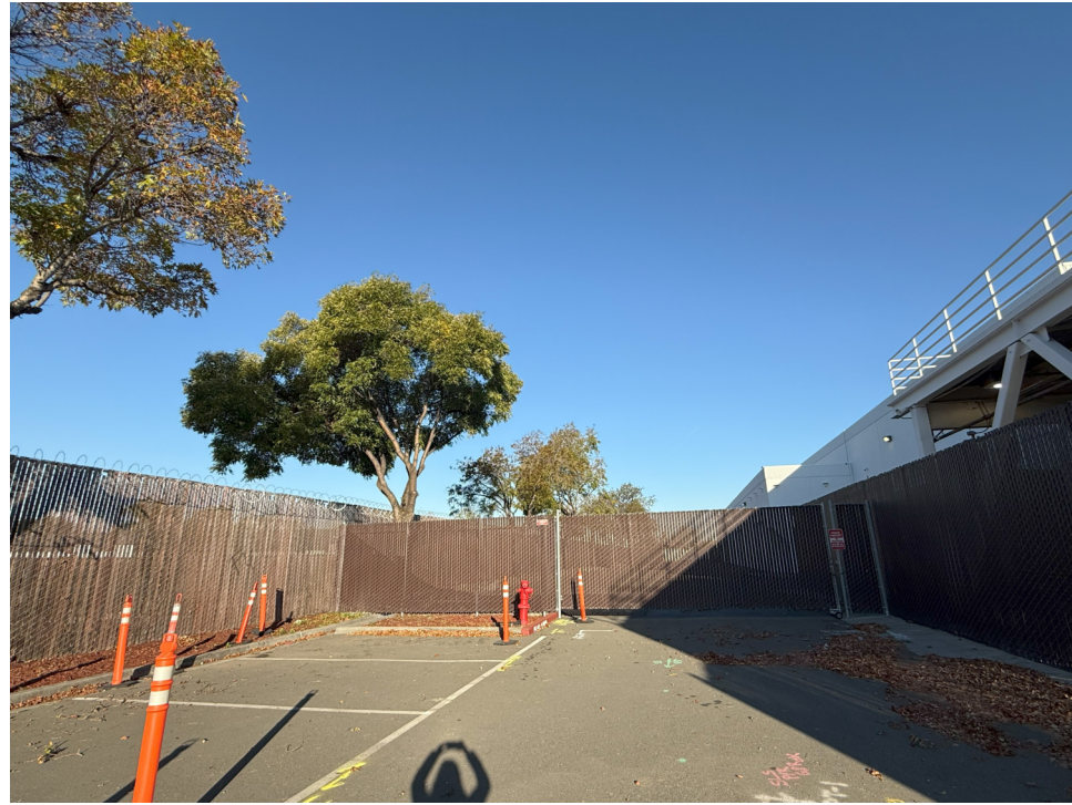
2 - VEHICULAR GATE TO SERVICE YARD (VIEW FROM PARKING LOT)
