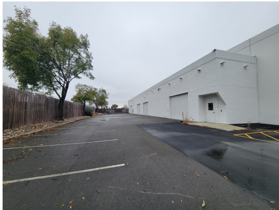
5 - VIEW FROM SERVICE YARD LOOKING NORTHWEST
