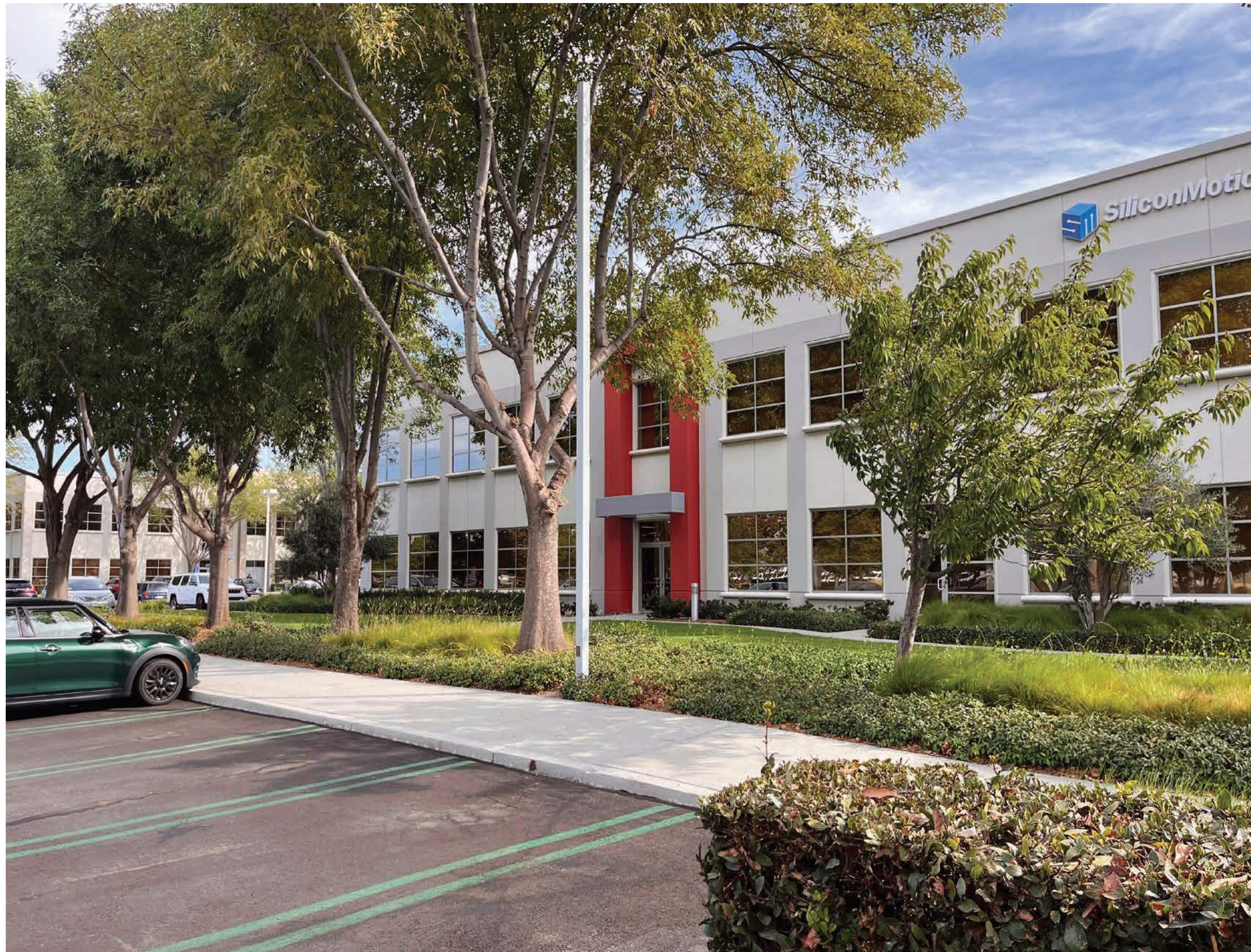
BEFORE: 690 BUILDING - WEST SIDE
