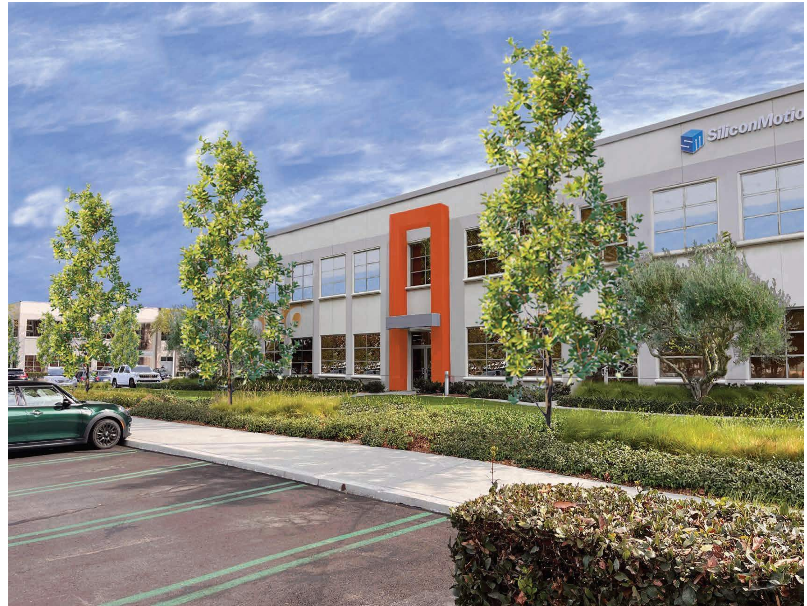
AFTER: 690 BUILDING - WEST SIDE
