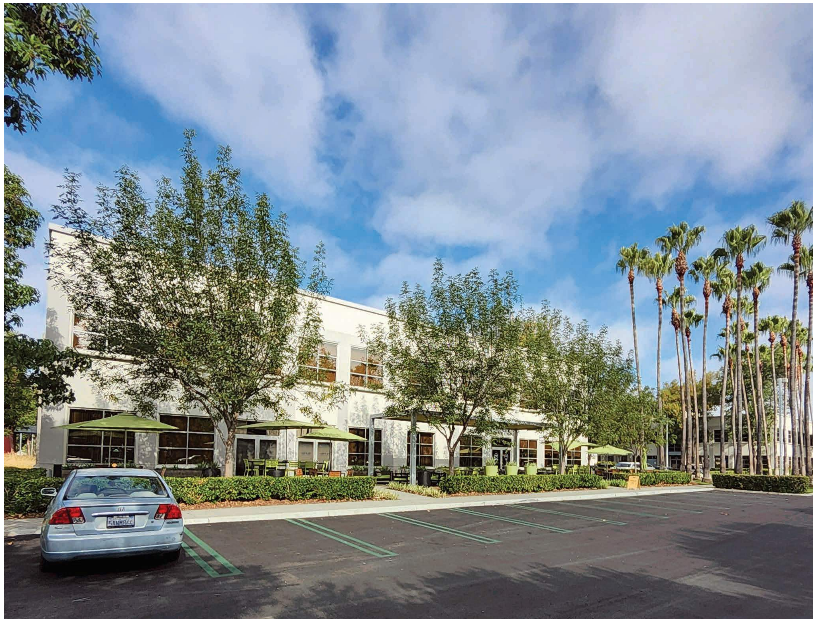
BEFORE: 690 BUILDING - EAST SIDE
