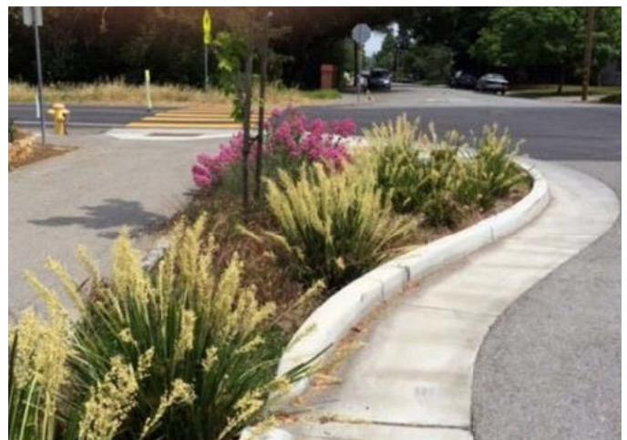
Figure 7-3 Stormwater Curb Extension, Los Altos
