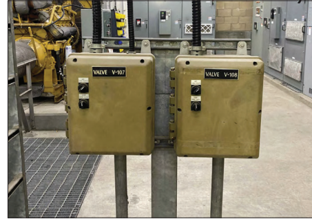
TYPICAL CONTROL STATION FOR VALVE 106, 107 AND 108
