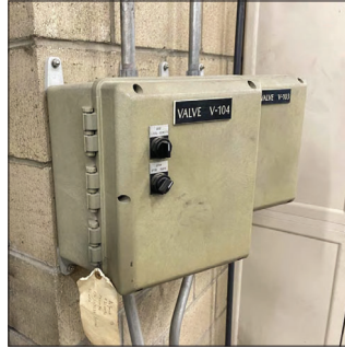
TYPICAL CONTROL STATION FOR VALVE 103, 104 AND 105
