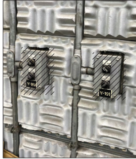
TYPICAL CONTROL STATIONS FOR VALVE 100, 101 AND 102 DEMO
