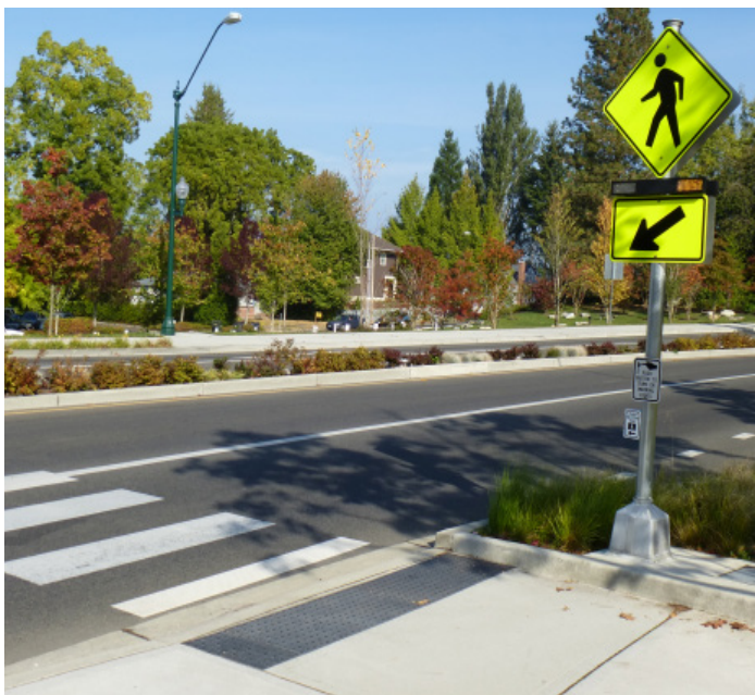
A rectangular rapid-flashing beacon (RRFB).
