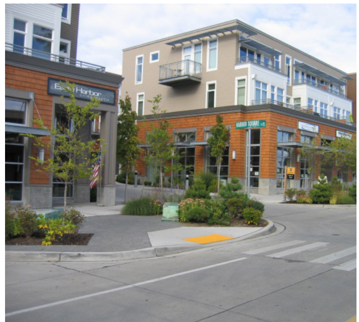
A planted curb extension at an intersection.
