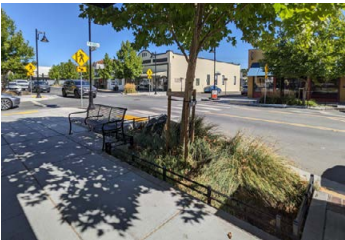
Examples of stormwater tree well filters located in the amenity zone of a sidewalk.
