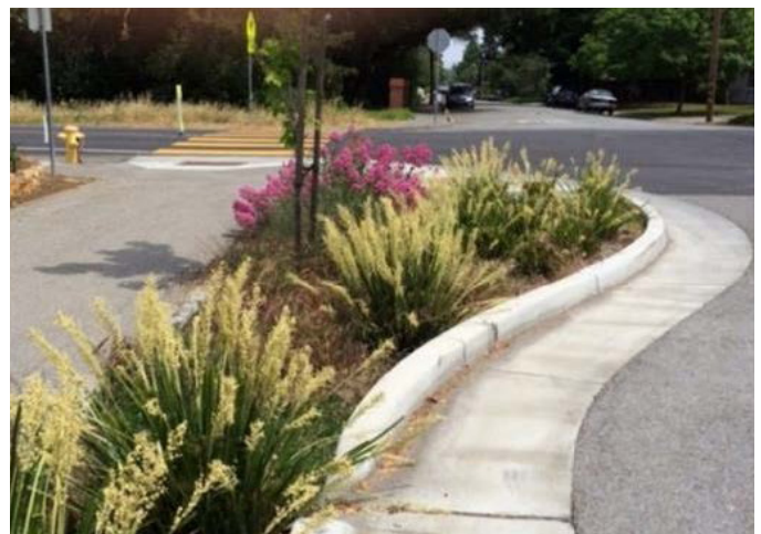
Figure 7-3 Stormwater Curb Extension, Los Altos
