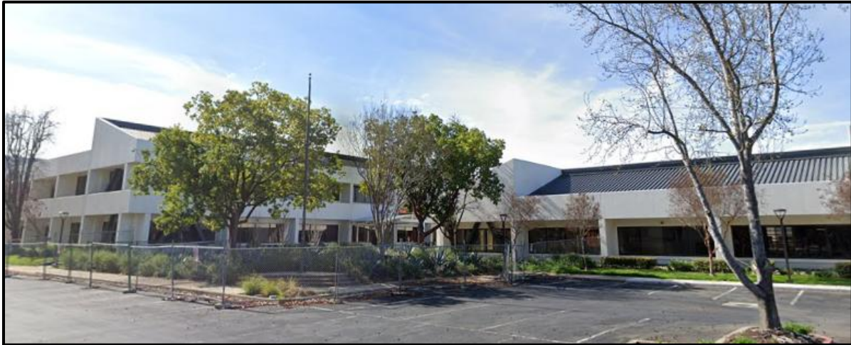
Figure 2: Partial View of Existing Onsite Buildings
