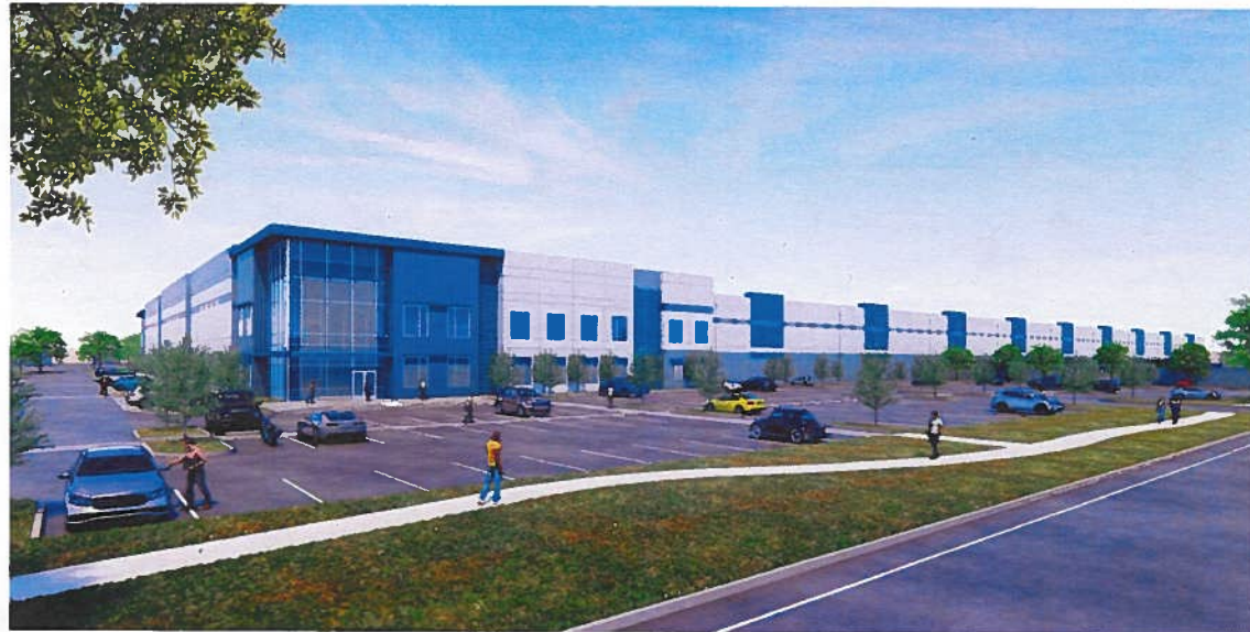
SOUTHEAST CORNER ENTRY FROM GIBRALTAR
