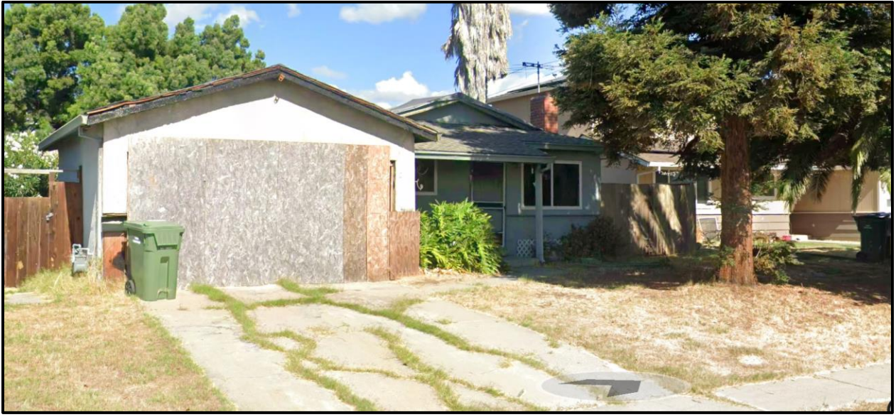
Figure 6: Previous Front Façade of 287 Duarte Ct.
