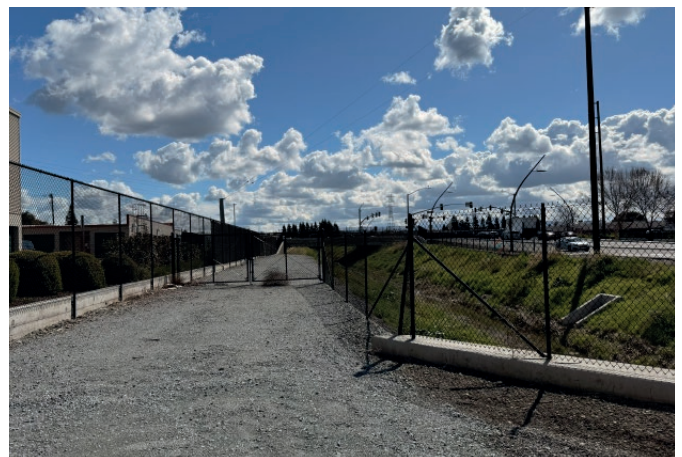
Fig. 2.12 - South View of Maintenance Access Path along Berryessa Creek North of Montague Expressway
