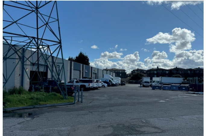
Fig. 2.4 - View of Private Property from S. Milpitas Boulevard
