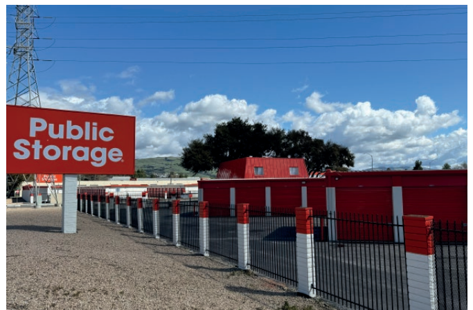
Fig. 2.8 - View of Public Storage Property from Montague Expressway
