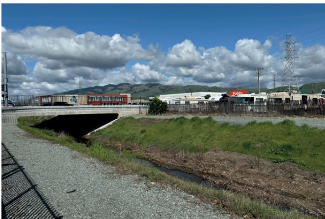
Fig. 2.7 - North View of Berryessa Creek at S. Milpitas Boulevard and Montague Expressway Intersection
