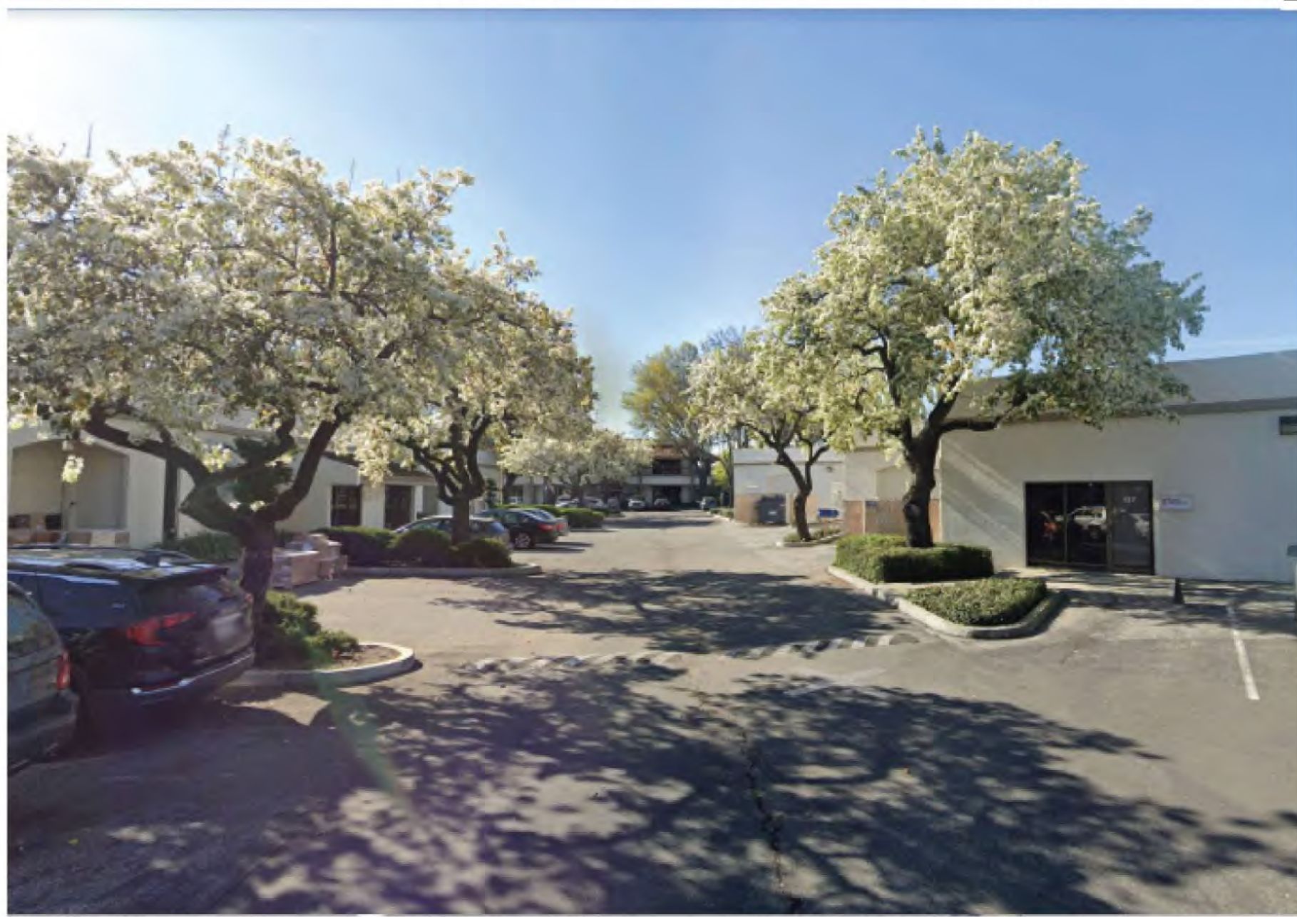
EXISTING SITE CONDITION - LOOKING SOUTH 5
