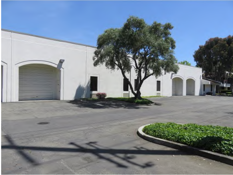
West façade, view facing east (ARG, April 2023).
