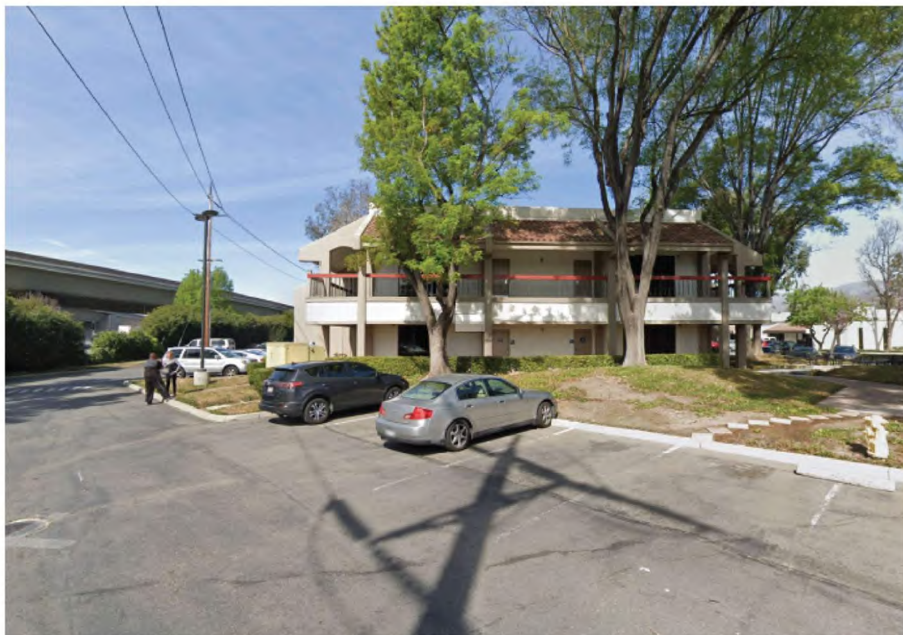
EXISTING SITE CONDITION - LOOKING NORTH 3
