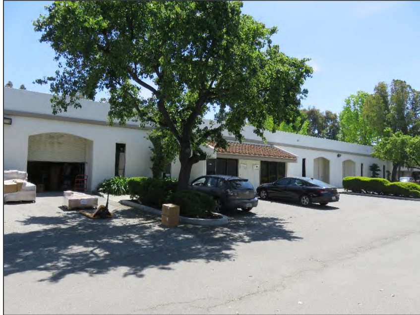
North façade, view facing south (ARG, April 2023).
