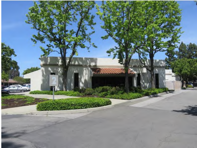
South façade with band of six fixed full-height windows, view facing north (ARG, April 2023).
