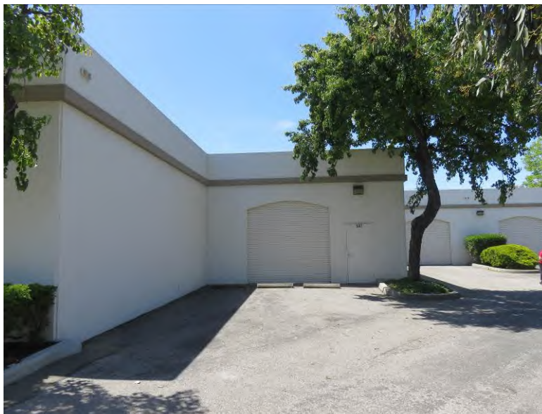
Industrial rolling service doors along winged east façade, view facing west (ARG, April 2023).
