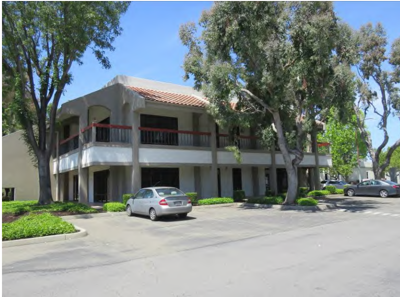
South façade, view facing north (ARG, April 2023).
