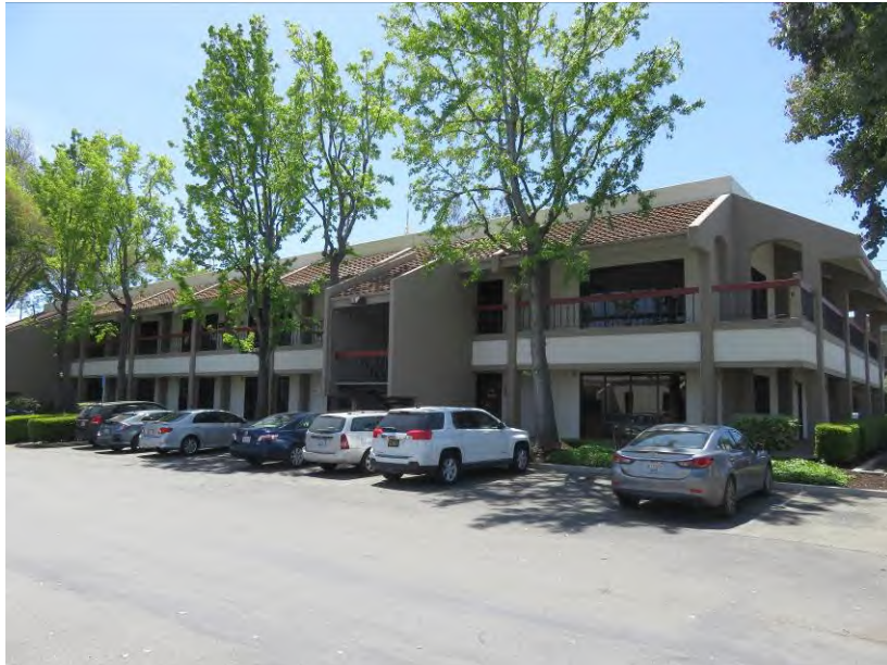
East façade, view facing west (ARG, April 2023).
