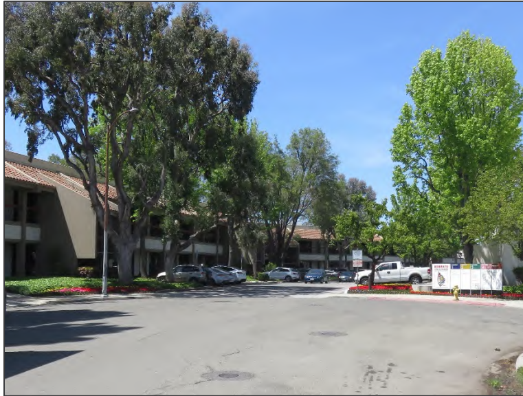
Overview of Calaveras Business Center from Valley Way cul-de-sac, view facing northwest (ARG, April 2023).
