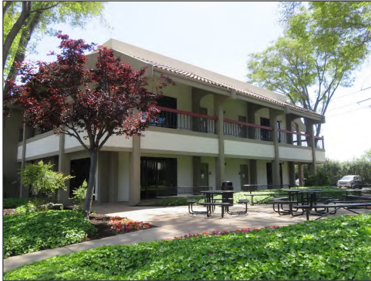
View of Building 3 and adjacent landscaping, including concrete patio area, view facing south-southeast (ARG, April 2023).
