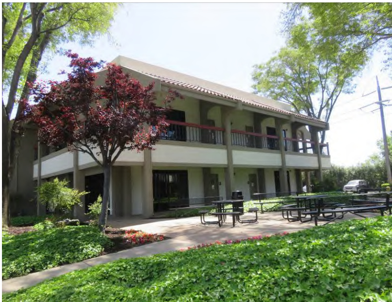
North façade and picnic area, view facing south (ARG, April 2023).
