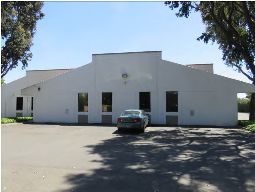
South façade, view facing north (ARG, April 2023).
