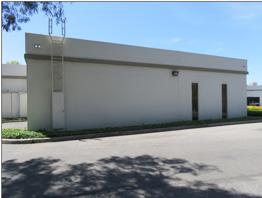
East façade, view facing west (ARG, April 2023).
