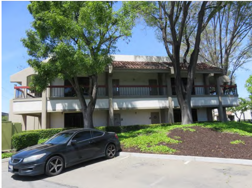
South façade, view facing north (ARG, April 2023).
