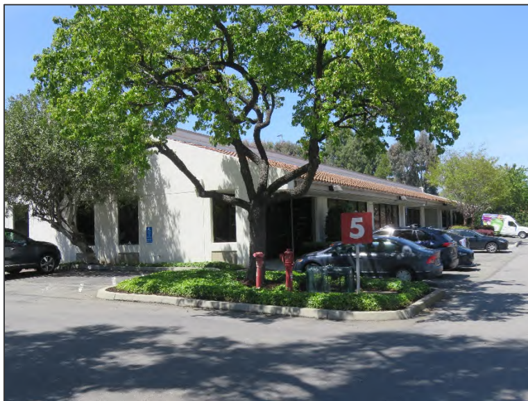
View of Building 5 and adjacent landscaping, parking, signage, and utilities, view facing northwest (ARG, April 2023).
