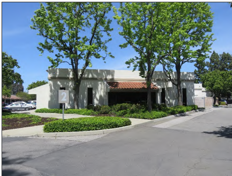
View of Building 2 and adjacent walkways and planting beds, view facing north-northwest (ARG, April 2023).
