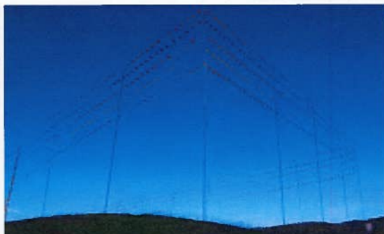
STORY POLES INSTALLED AT SETBACK LINES AND CONTINUED INTO CRESTRLINE ZONE OF PROTECTION.
