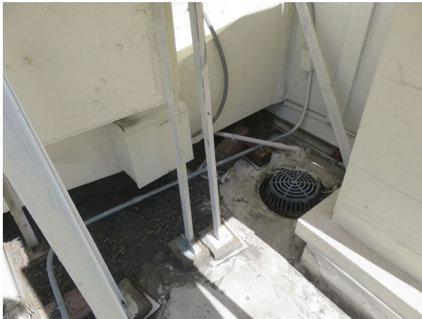
Roof drain near AC-5
